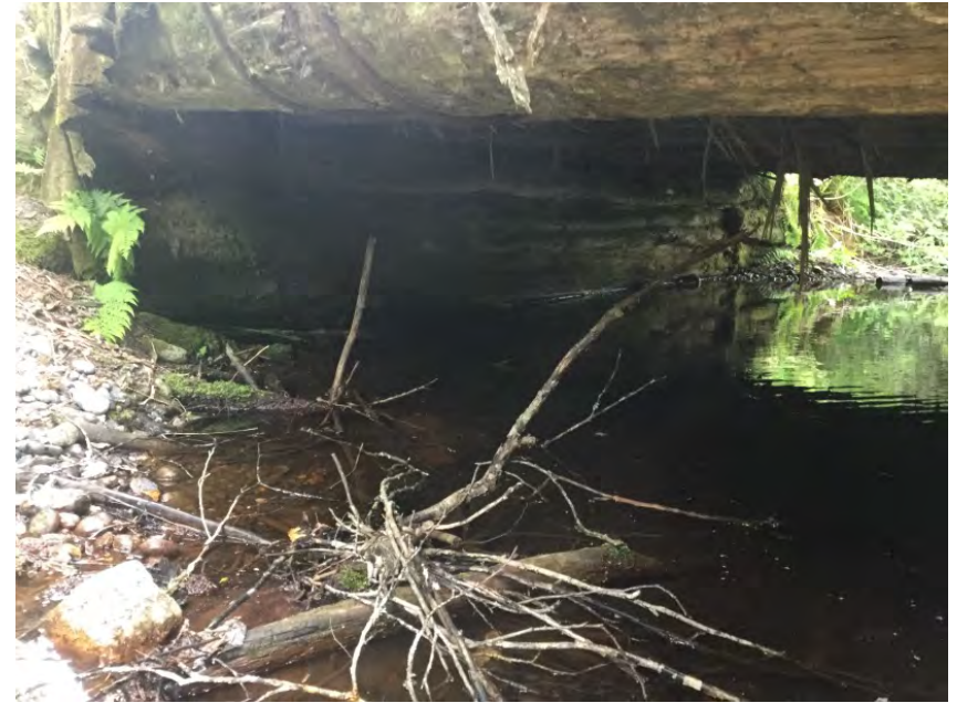
Left Bank Abutment when facing downstream
