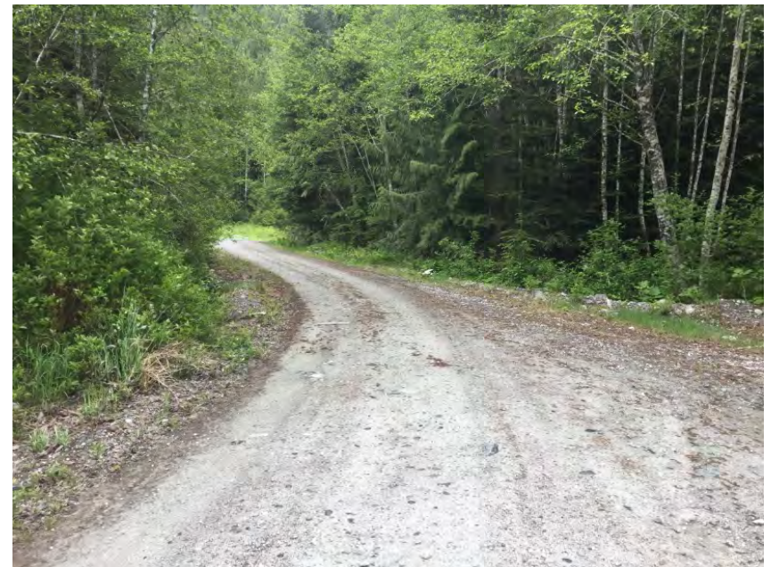
Approach from Right Bank when facing downstream
