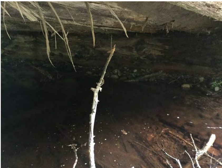
Right Bank Abutment when facing downstream
